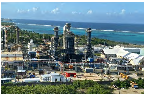
The USVI Water and Power Authority (WAPA), St. Croix, USVI. Photo Source: VI Consortium
